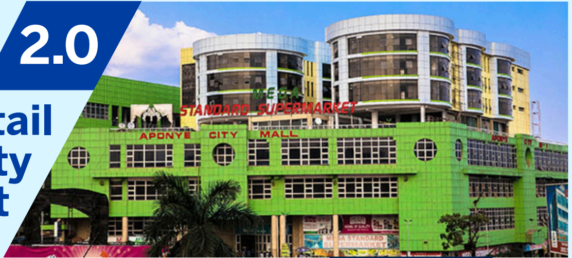
Aponye City Mall - Burton Street
